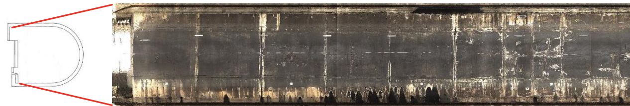
Image of tunnel lining captured for inspection
