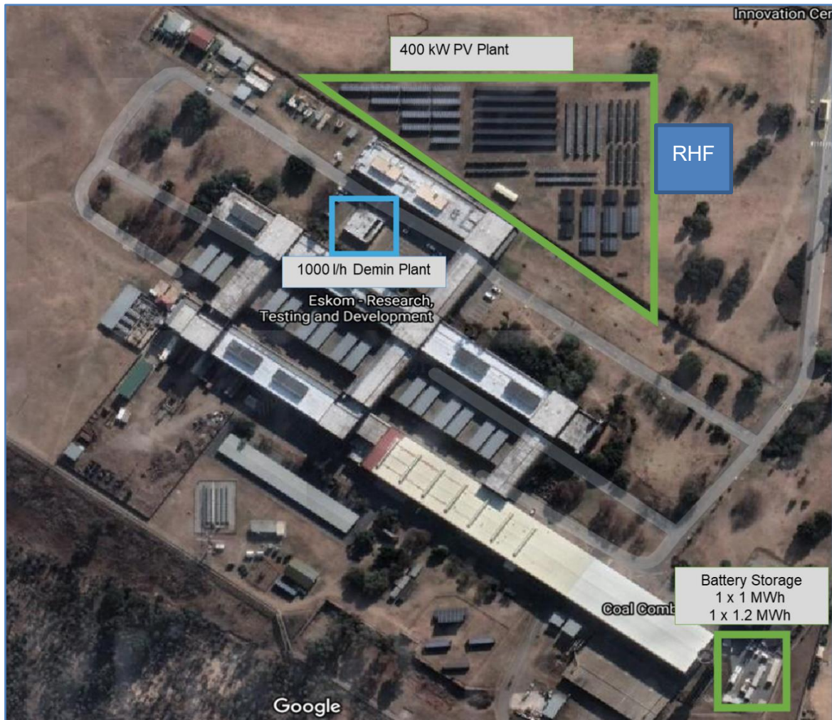
Figure 3: ERIC, RT&D premises at Rosherville for RHF implementation
