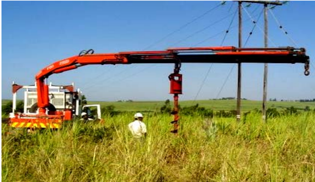
Figure 1: Auger secured on the boom
