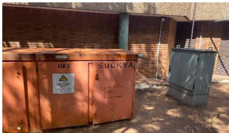
Figure 3: Security Office Mini-Substation 11kV Meter Kiosk
