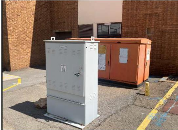
Figure 5: Tulip Substation 5 Meter Kiosk
