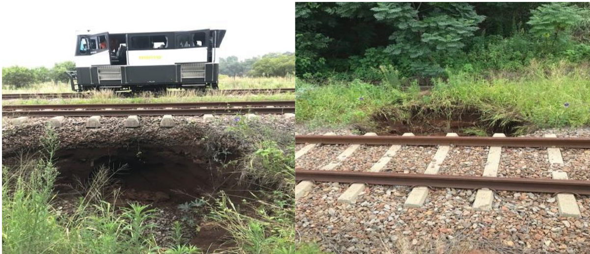
Figure 1: The re-occurrence of sinkholes in the Centurion station area
