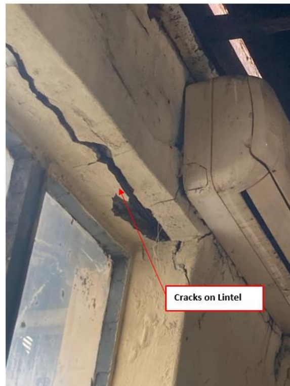
Figure 5: Wall Cracks Close to Windows
