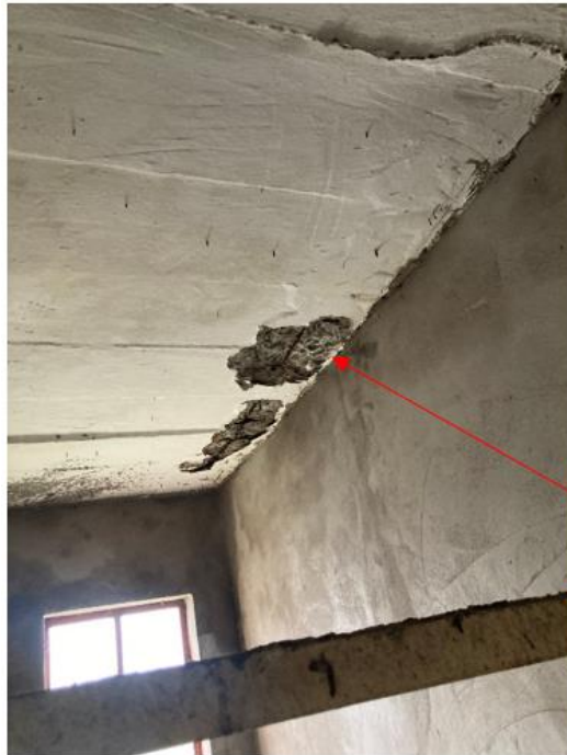
Concrete Spalling on Rood Slab Soffit
