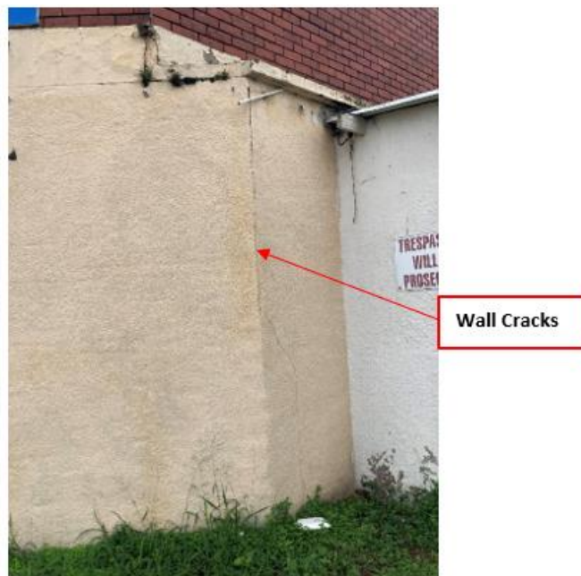
Figure 9: Exterior Cracks
