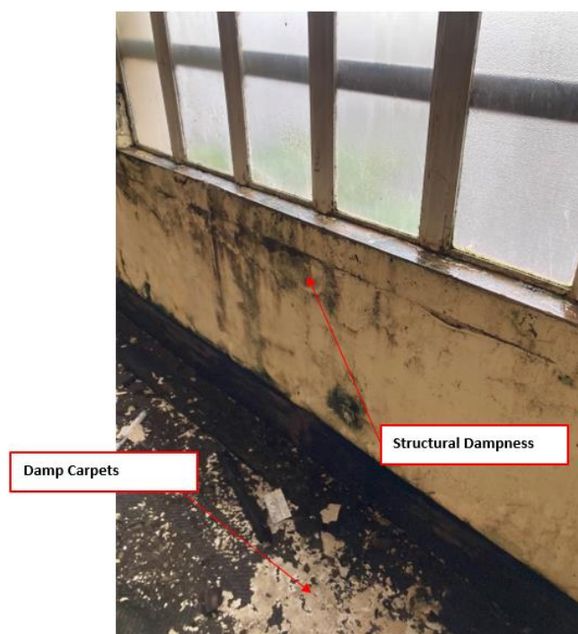
Figure 6: Wall Dampness
