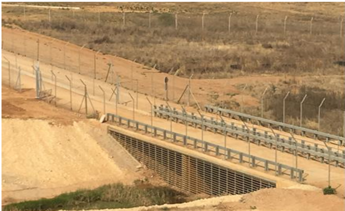
Figure 7: Security Grid Arrangement (Culvert/Bridge Crossing)
