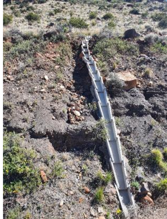
N01-09 km 1+84 Chute Failure - erosion
