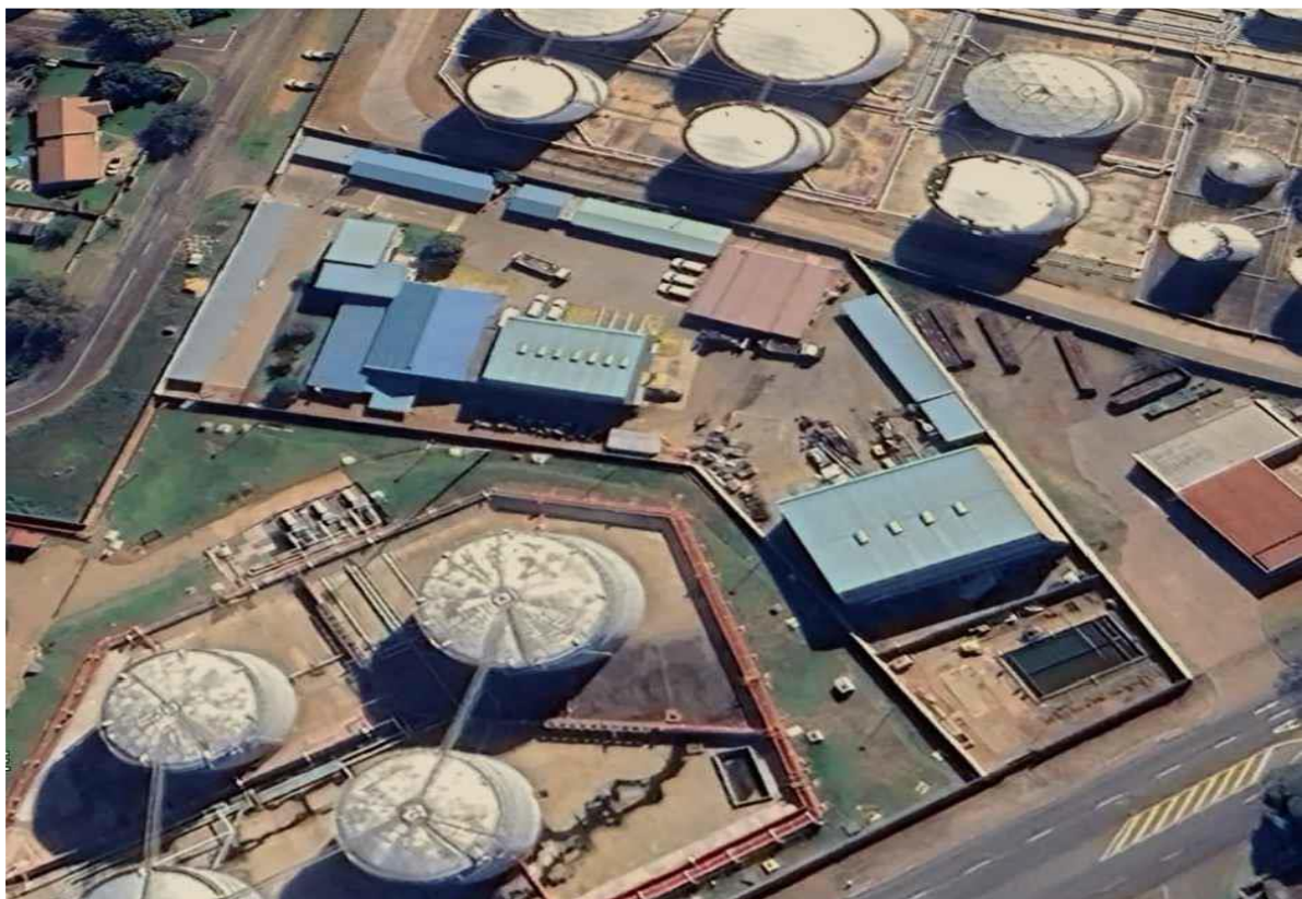
Figure 1: Aerial View of the Alrode Depot Facilities
