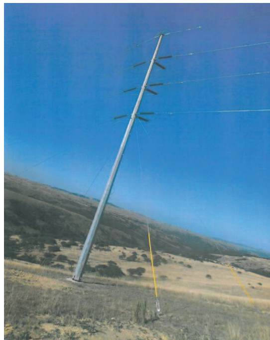
Figure 4 : Guyed monopole strain structure (D-DT-7645)
