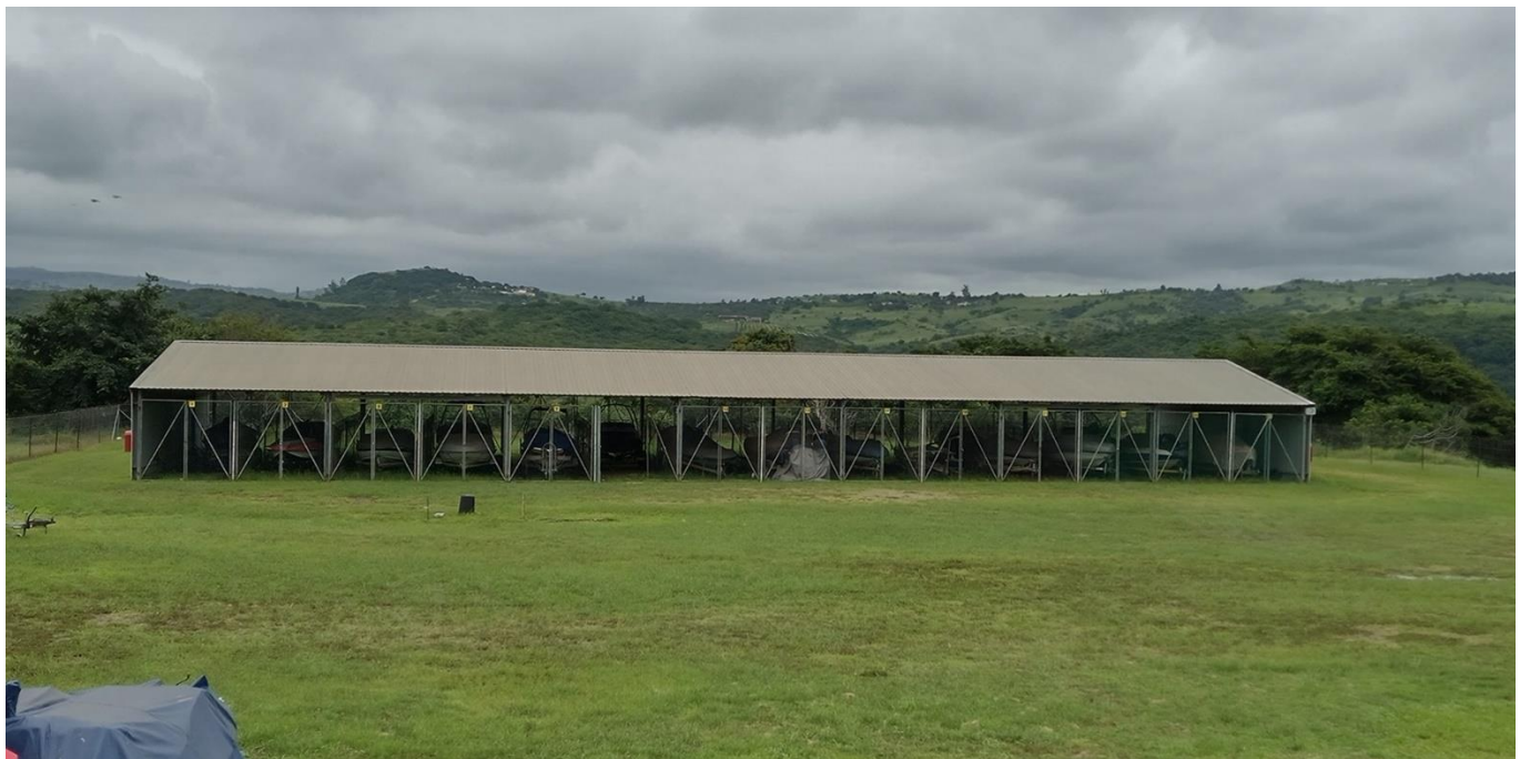
Figure 2: Showing existing closed boat lockers at Hazelmere Dam and Resort.
