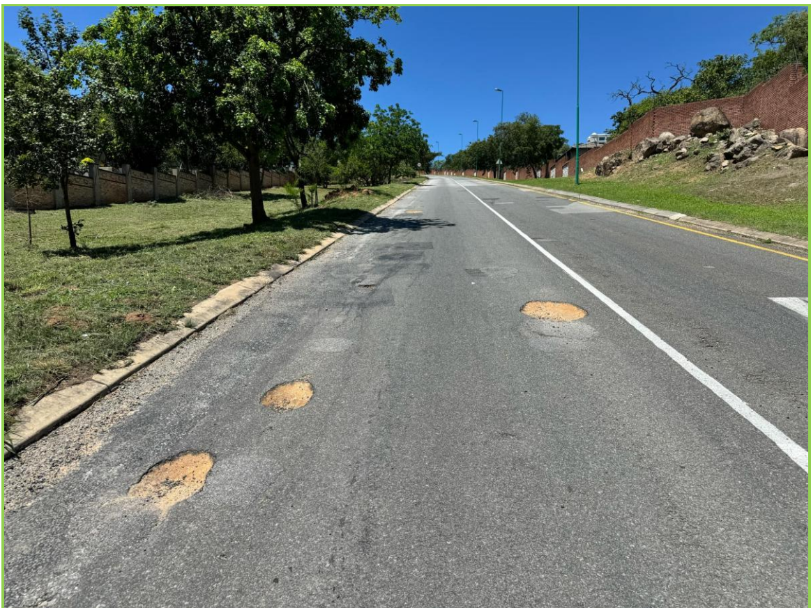
Figure 3: Severe cracks and defects on the old pavement caused by heavy vehicles
