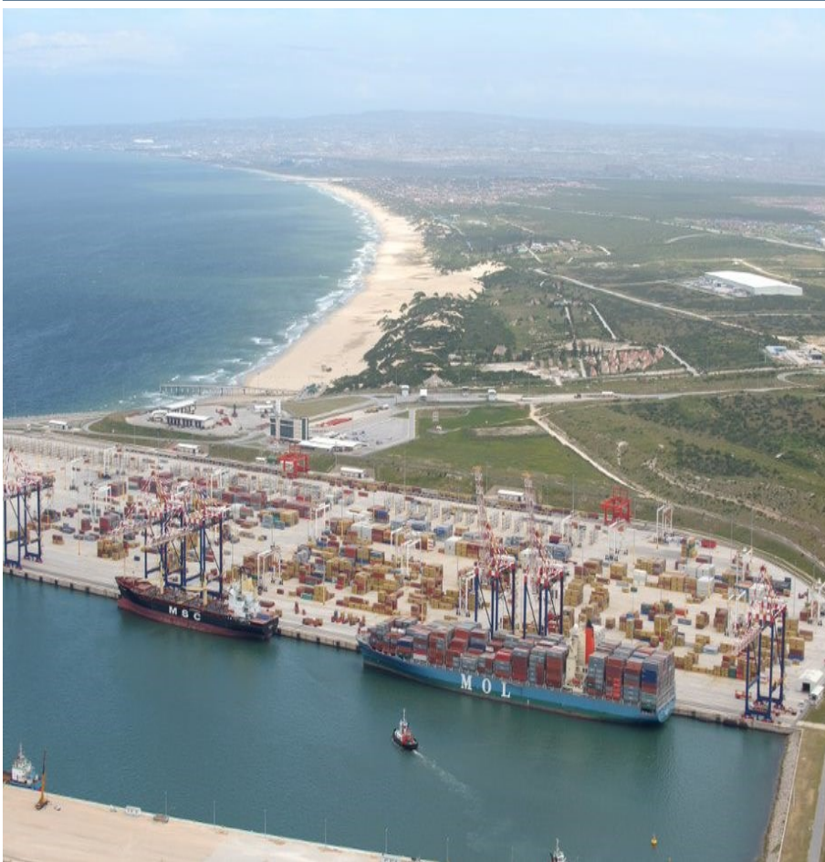
Picture: Port of Ngqura
