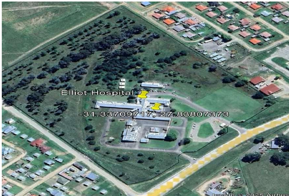
ELLIOT HOSPITAL AERIAL VIEW (SOURCE GOOGLE EARTH)
