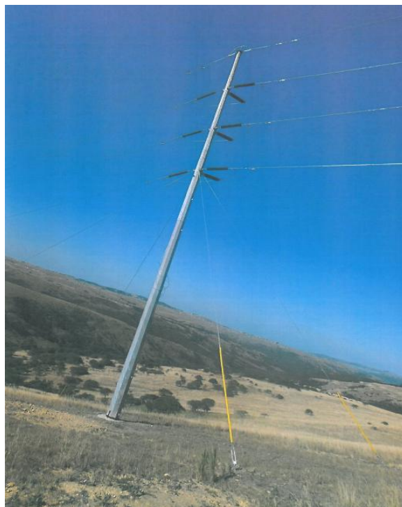
Figure 4 : Guyed monopole strain structure (D-DT-7645)
