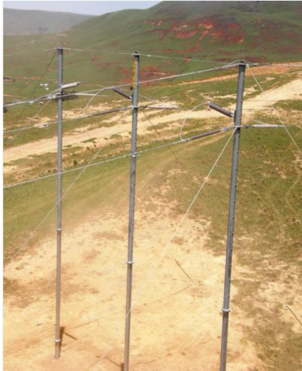
Figure-5 : Steel Trips monopole strain structure (D-DT-7618)
