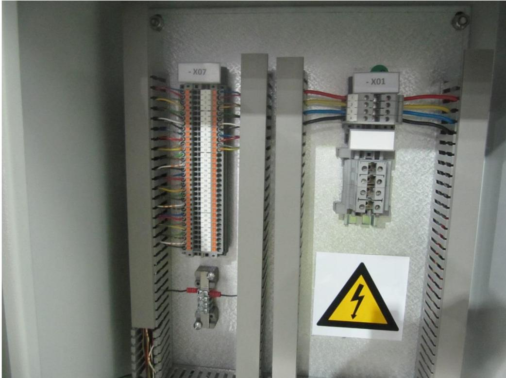
**Figure 8: Typical Internal Layout of a Splitter Box**
