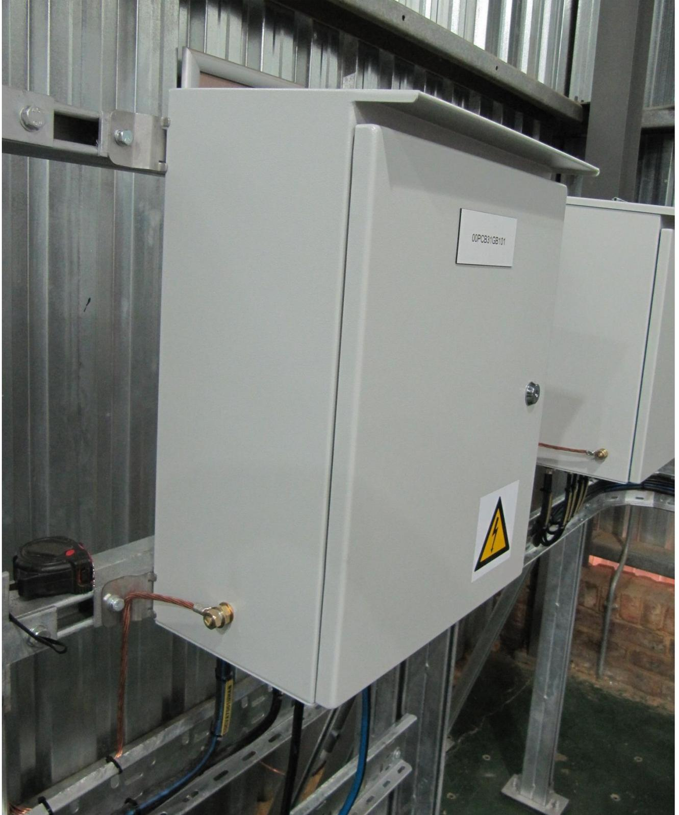
**Figure 7: Typical Field Junction Box.**
