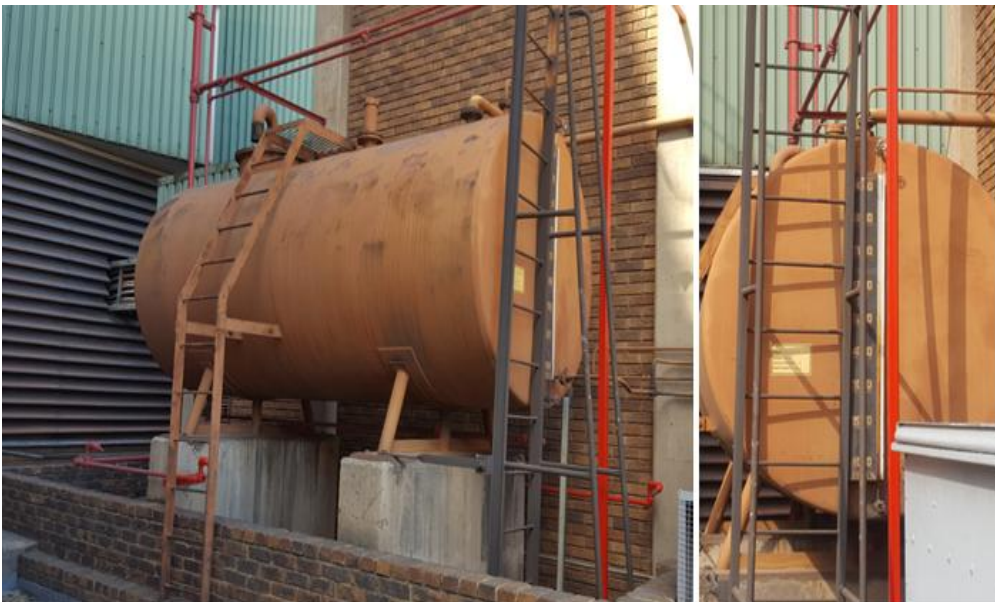
Figure 8: Diesel Storage Tank and Level Indication
