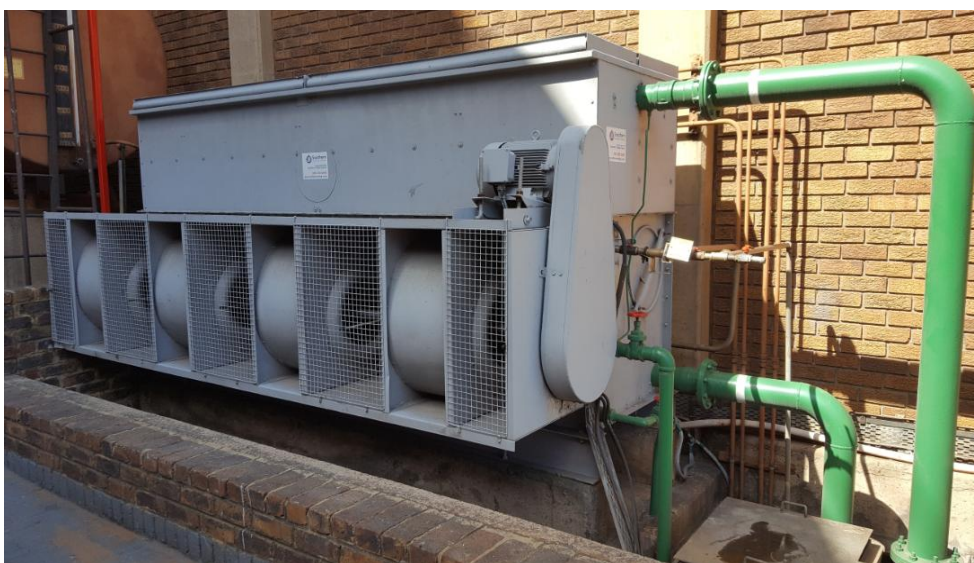
Figure 6: Cooling Tower
