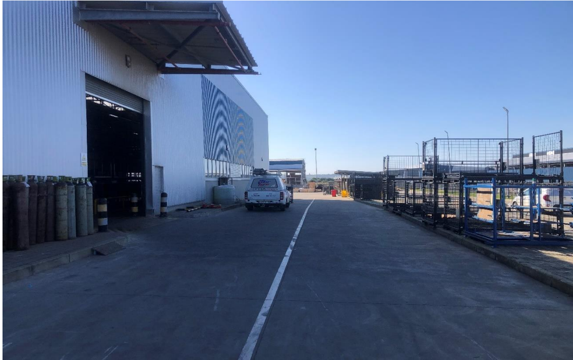
New enclosed dispatch canopy (site information ref 1)
