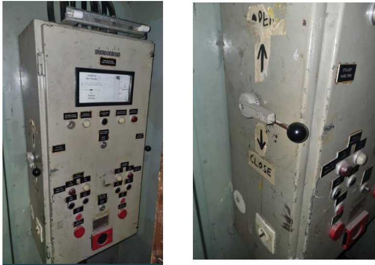
Pictures 16 & 17 – Stage level Control Panel
