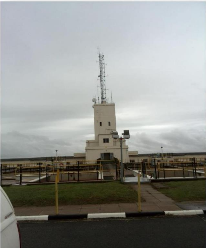
25M lattice tower on top of the Building
