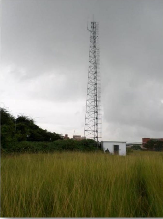
36M lattice tower
