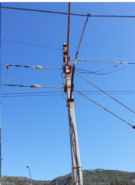
Figure 4: Rusty Small steel parts
