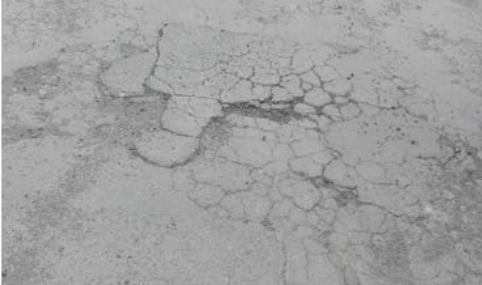
Figure 6: Crocodile Cracking
