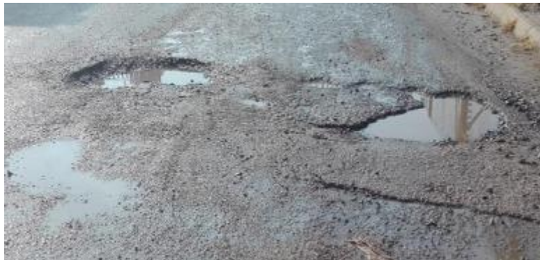
Figure 3: Potholes
