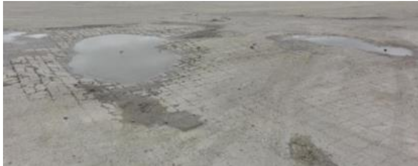
Figure 9: Settled Segmental Block Paving
