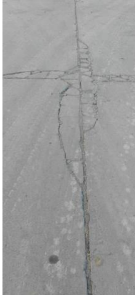
Figure 8: Rigid Pavement Damage
