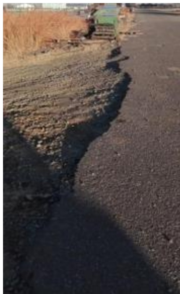
Figure 5: Edge Break Damage
