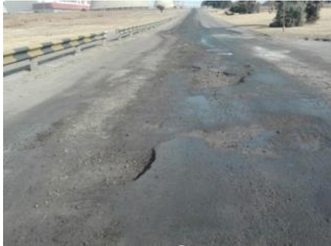
Figure 4: Pavement Failure
