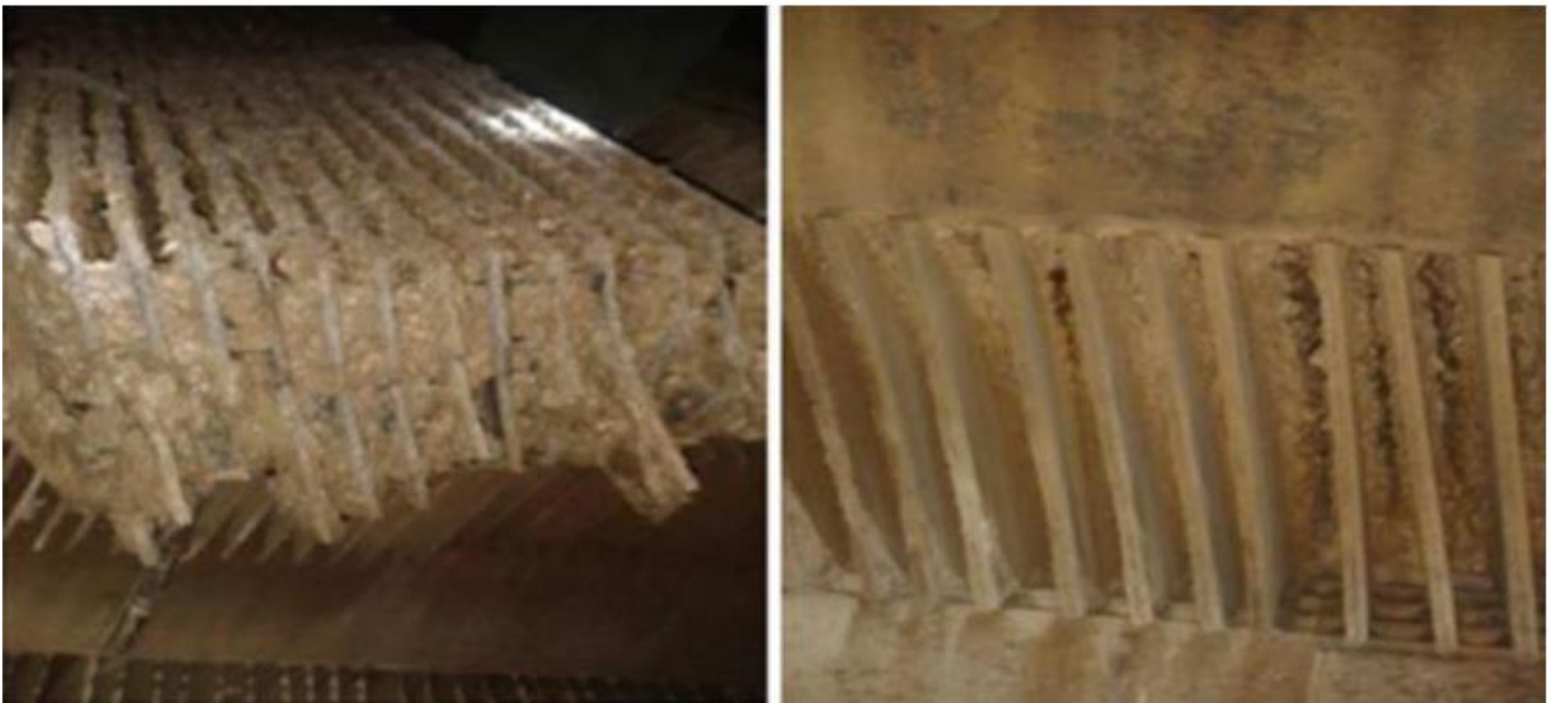
Figure 4: Side view of clogged asbestos fill at Tutuka PS
