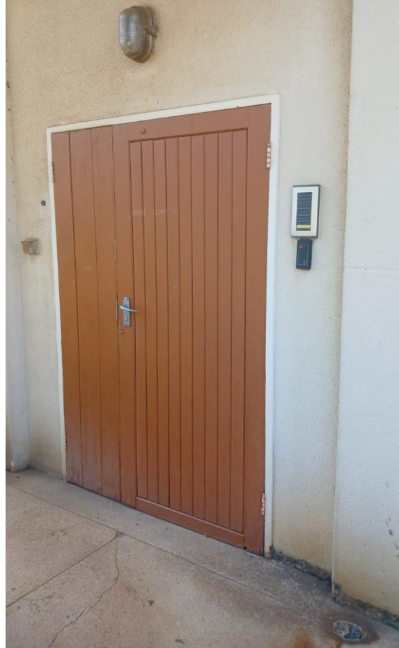
Current second stairs door
