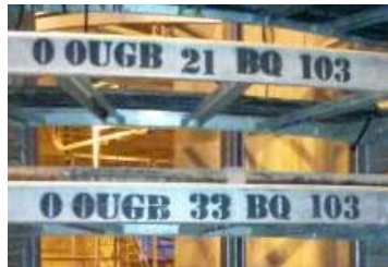
Figure 36: Cable rack/tray stencilled example
