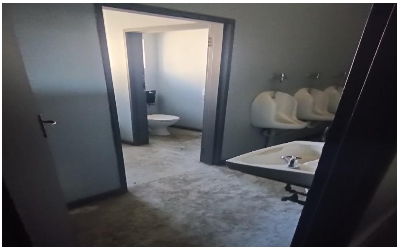
Ablution Facilities inside the Workshop
