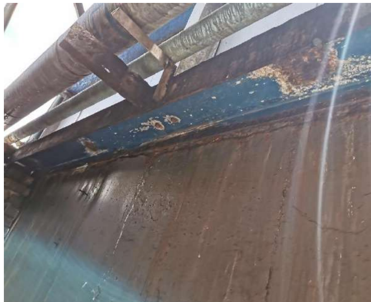
Figure 53: Pipe support beam rusted.
