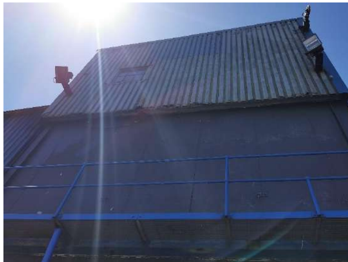
Figure 45: Sheeting and side girt rusted and in bad condition.
