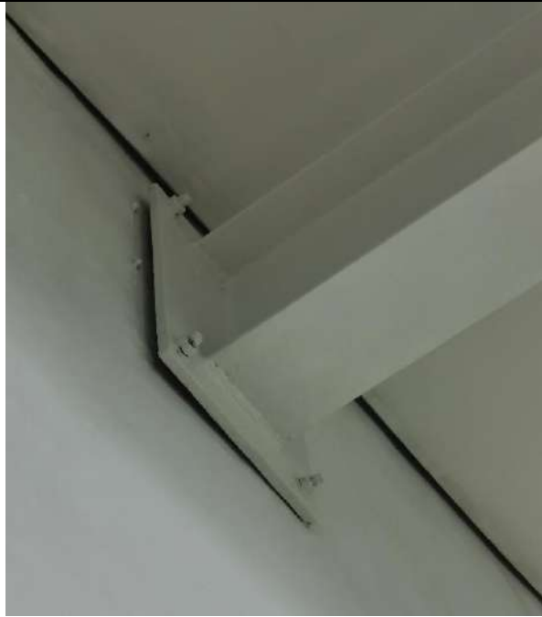
Figure 11: Gap between I-Beam baseplate and brick wall
