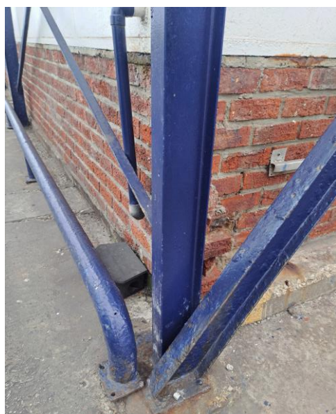
Figure 2: Treated members with traces of corrosion
