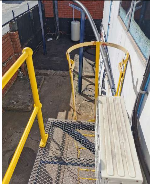
Figure 25: Cat-ladder not secured and there is a gap between cat-ladder and handrail.
