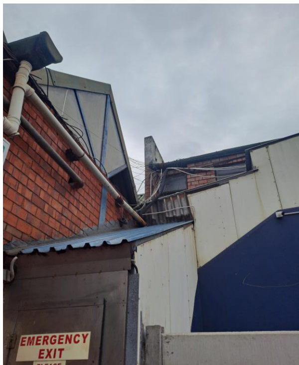
Figure 3: Missing roof side panel (triangle)
