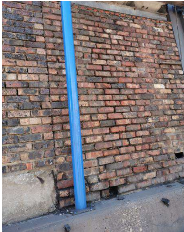
Figure 35: Fretting mortar on the north-western side of the building
