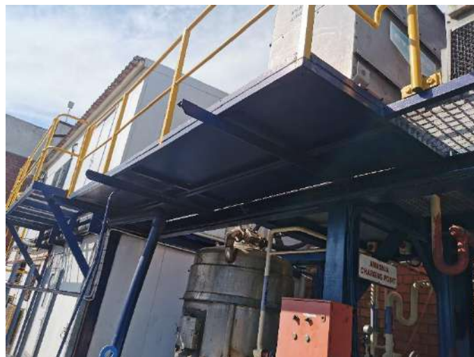
Figure 21: Evaporative condenser platform
