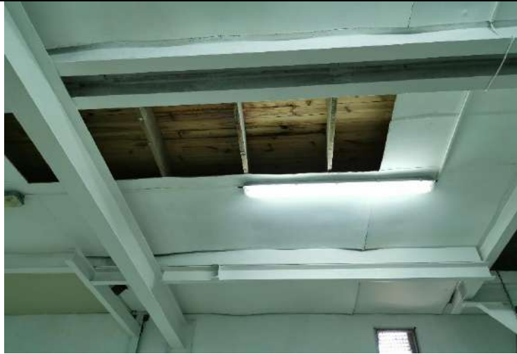
Figure 15: Timber rafters @ 635mm c/c and timber boarding
