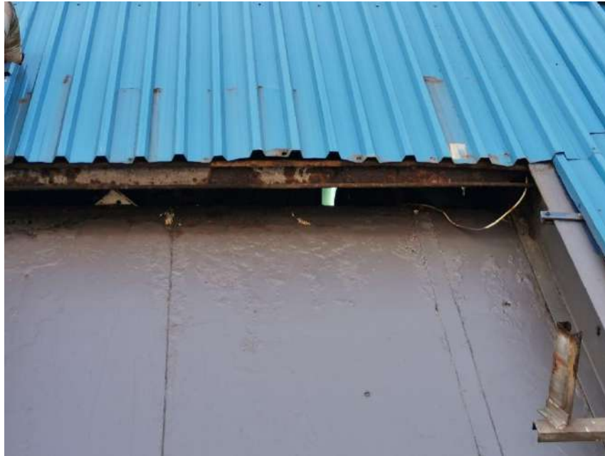
Figure 46: Sheeting and side girt rusted and in bad condition.
