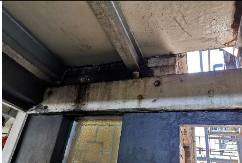
Figure 41: Timber beam at the back of brickwork supporting the steel beams
