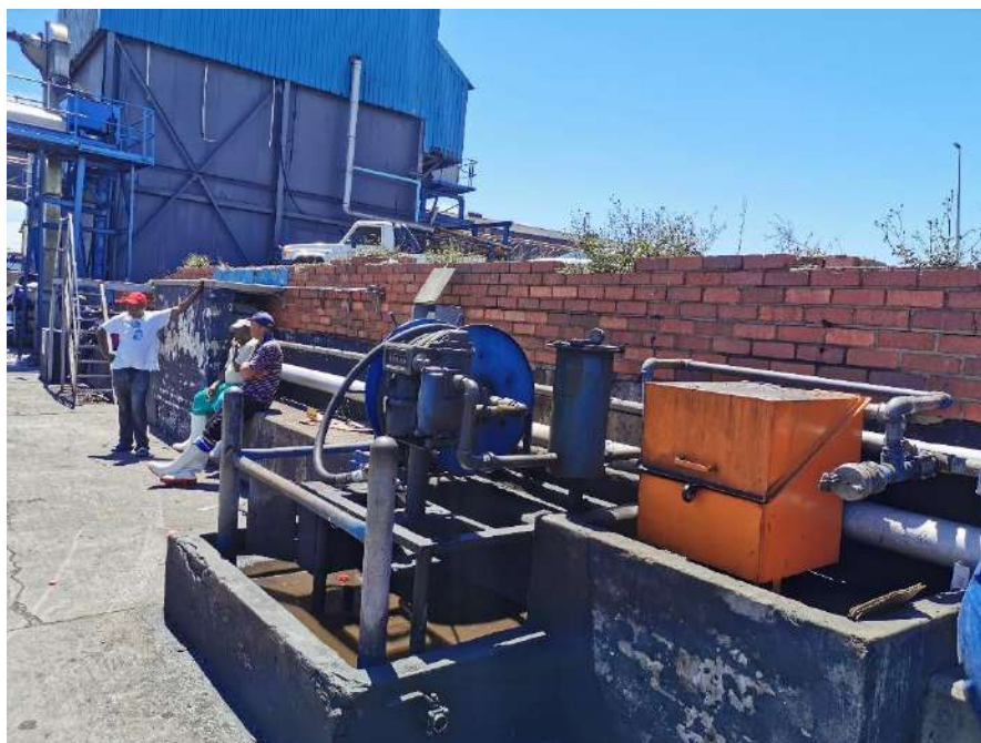
Figure 66: There is no handrail on top of the retaining wall
