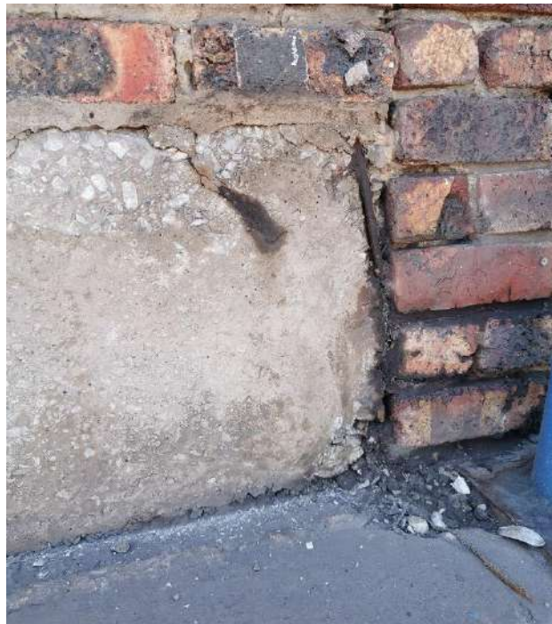
Figure 36: Spalled concrete on the north-western side of the building
