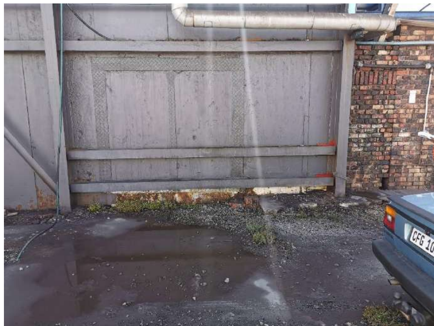
Figure 49: Iso panels rusted
