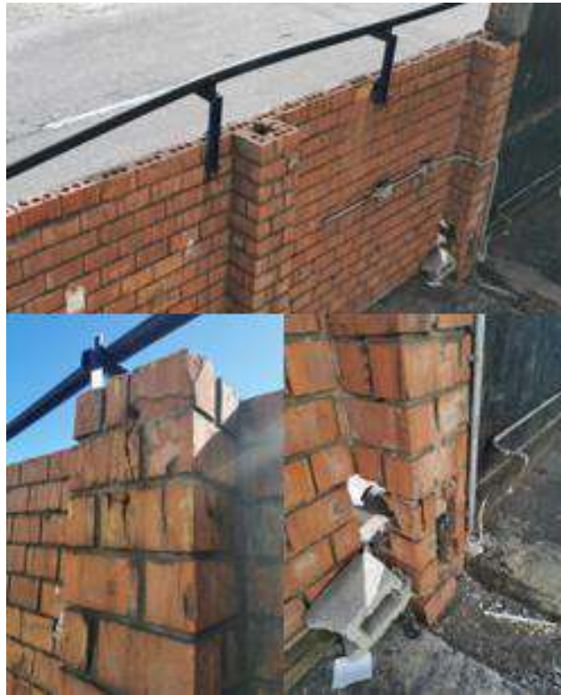
Figure 29: Damaged pillars to be replaced.
