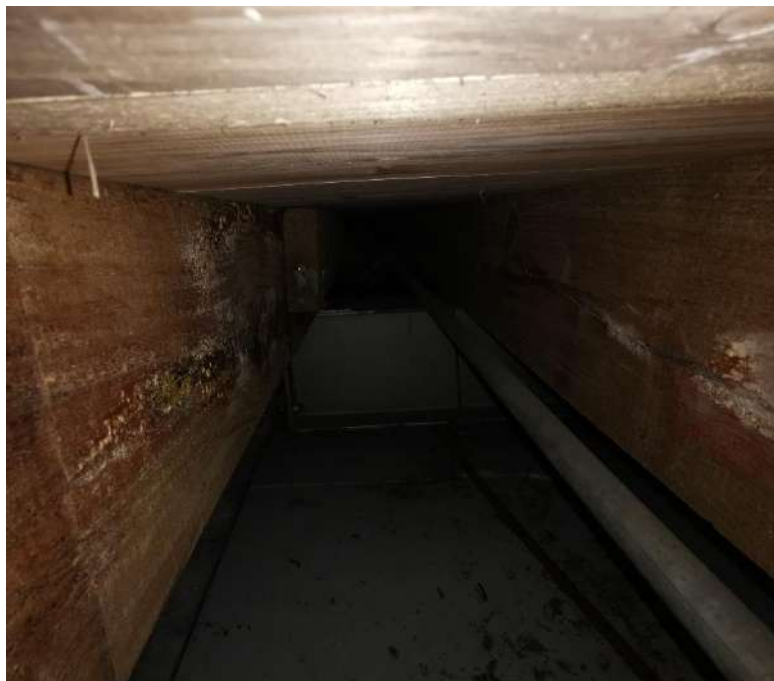
Figure 6: 76 x 228mm SAP rafters spaced at 415mm c/c
