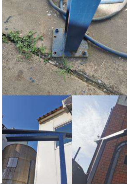
Figure 27: One baseplate with missing HD bolt and pipe to be secured to structure with aluminum straps
