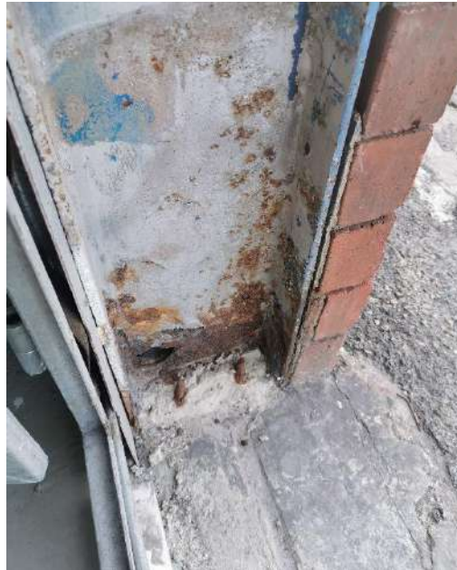
Figure 17: Rusted door steel stanchions
