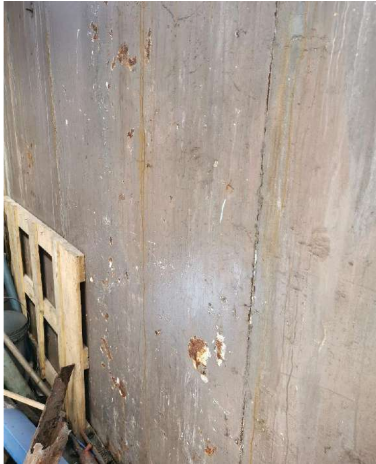
Figure 52: Rusted iso panels
