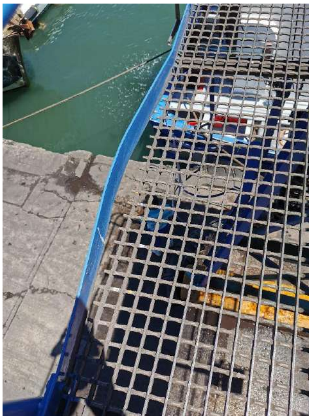
Figure 62: Kick plates buckling
