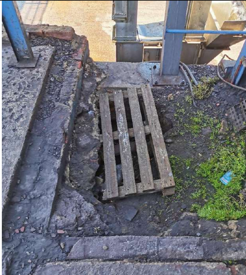
Figure 63: Hole must be filled with granular material
