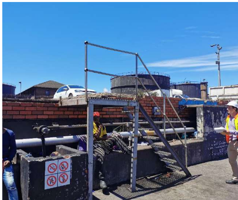
Figure 64: Unstable steel staircase with no handrail on one side.
