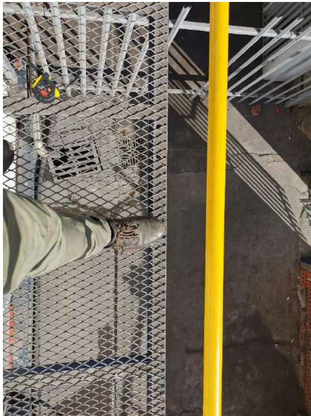
Figure 26: Expanded metal type mesh and no kick plates
