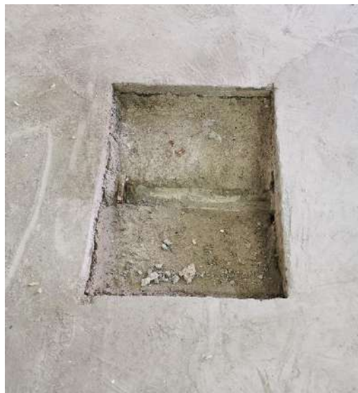
Figure 18: The floor drain has no cover
