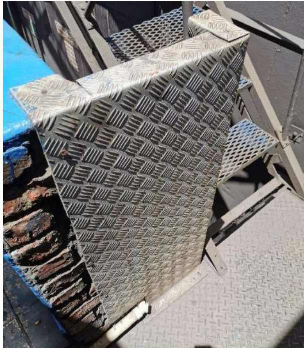
Figure 43: Aluminium panel to be secured properly
