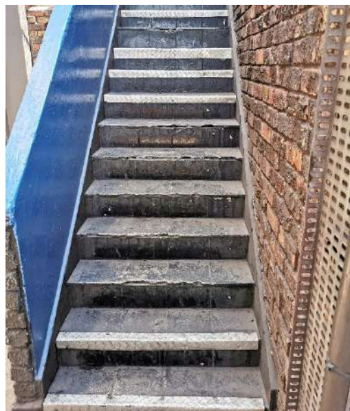
Figure 42: Aluminium strips missing on edges of stair treads
