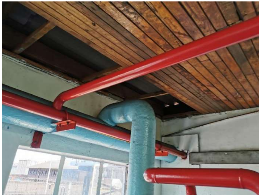
Figure 44: Damaged ceiling in plant room on first floor
