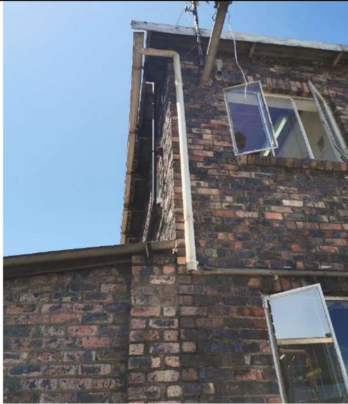
Figure 39: Inadequate roof drainage
