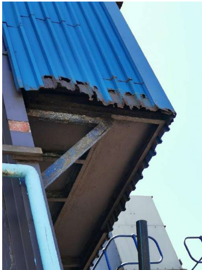
Figure 47: Sheeting and side girt rusted and in bad condition.
