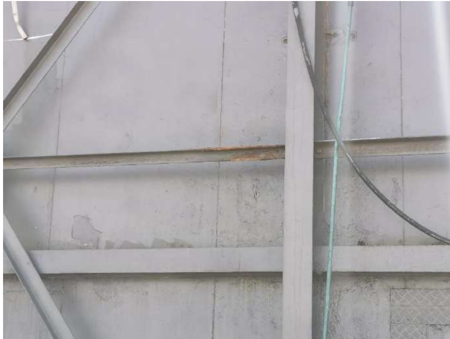
Figure 48: Some bracing members are rusted.
