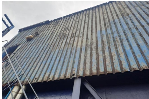
Figure 6: Severely corroded vertical sheeting
