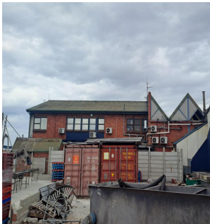
Figure 4: Roof sheeting requires painting
