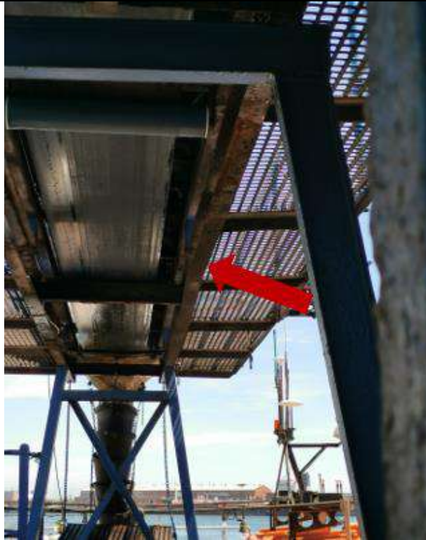
Figure 61: Rusted beam buckling out of plane.
