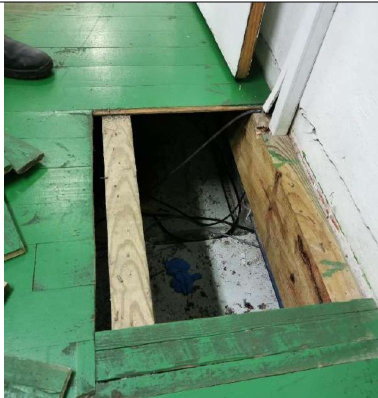
Figure 5: Section of floor boarding cut to inspect timber rafters
