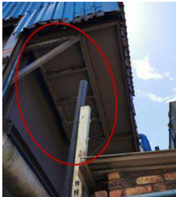
Figure 51: Platform support structure rusted
