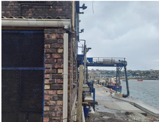
Figure 5: Dittached downpipe from the eave
