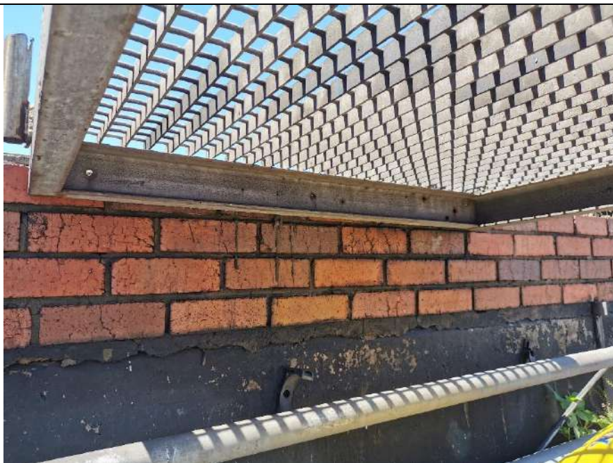
Figure 65: Steel staircase landing not bolted to brick wall
