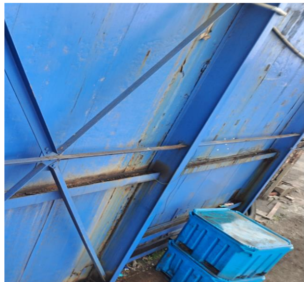
Figure 8: Water stuck in the I beam causing further corrosion
