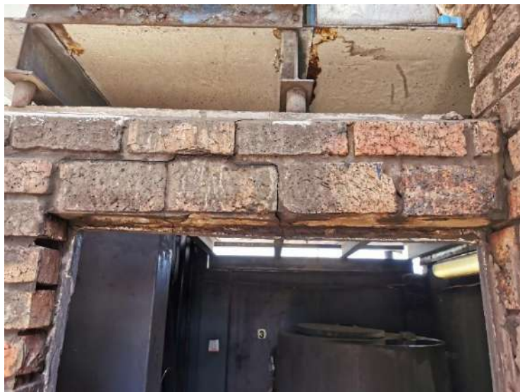
Figure 40: No lintel over opening and cracked brickwork
