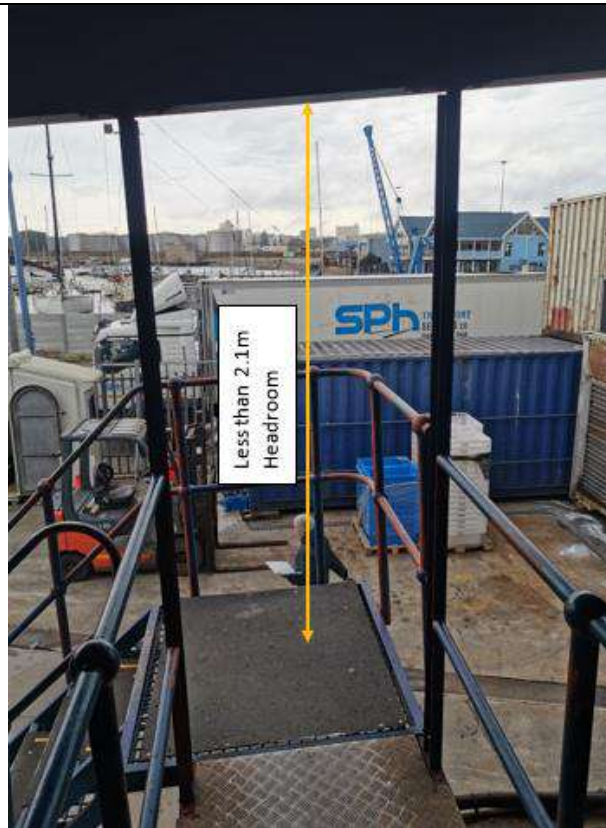
Figure 30: Headroom less than 2.1m
