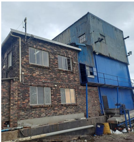
Figure 7: Missing downpipe
