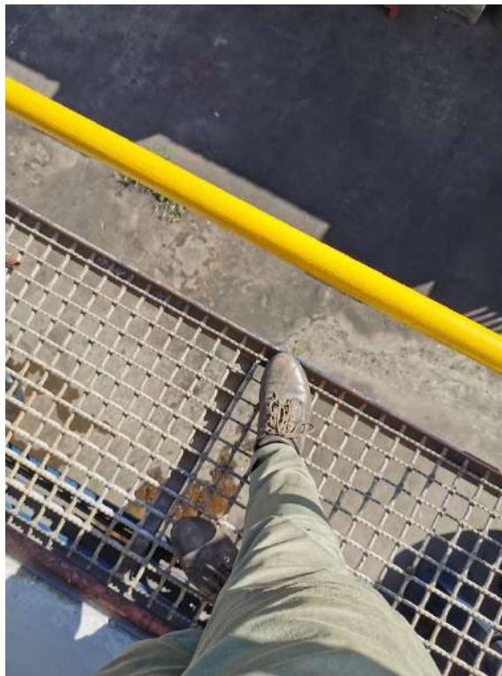
Figure 23: No kick plates on the edge of the walkway
