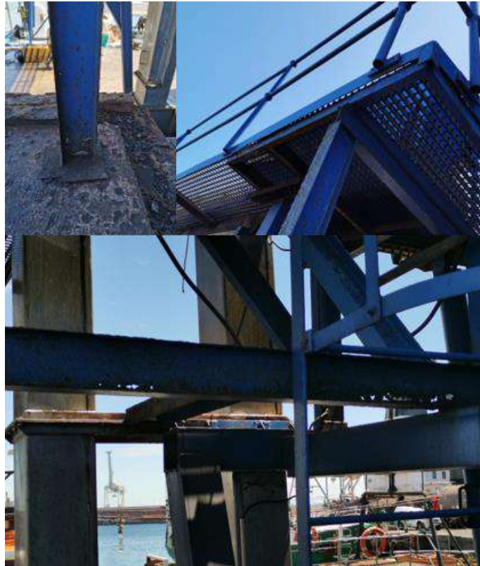
Figure 60: Rusty members of ice delivery structure
