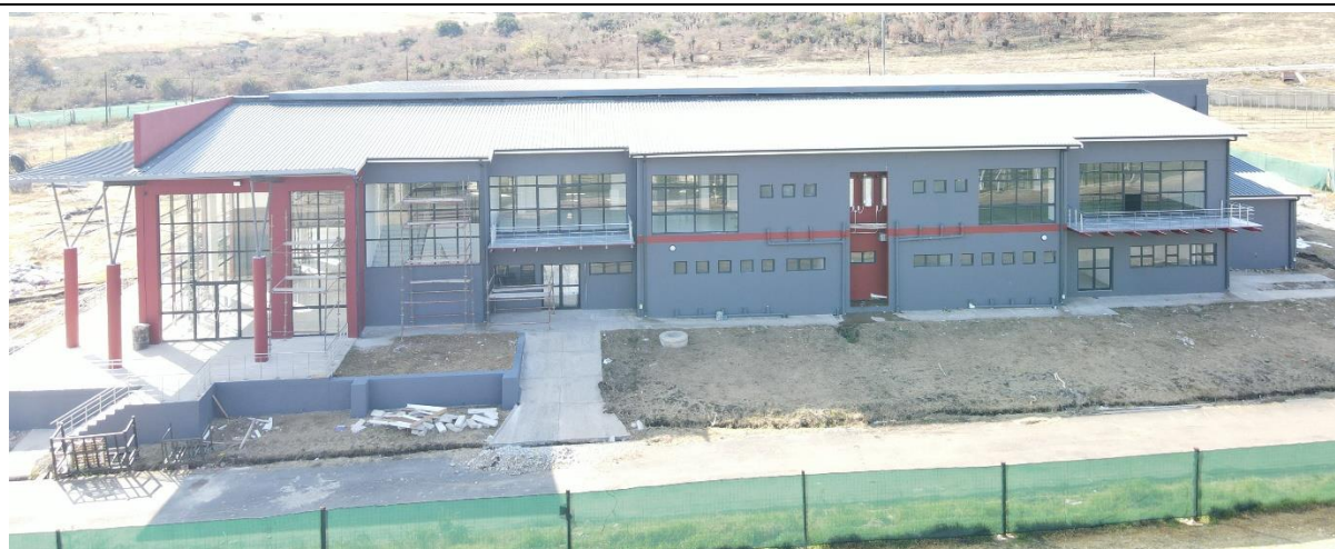
Front View of the MPC Building. Construction of concrete drains and general landscaping around the building structure is required.
