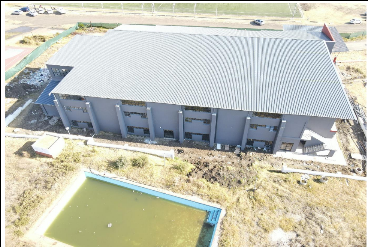
Rear View of the MPC : Construction of ramp for disabled is required to provide access to the swimming. Construction of concrete paving of walkways, concrete drains and general landscaping around the building structure is required.
