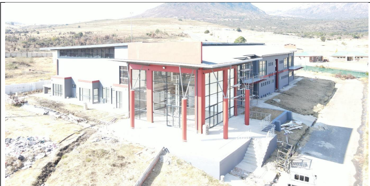
Side View of the MPC Building. Construction of concrete paving of walkways, concrete drains and general landscaping around the building structure is required.
