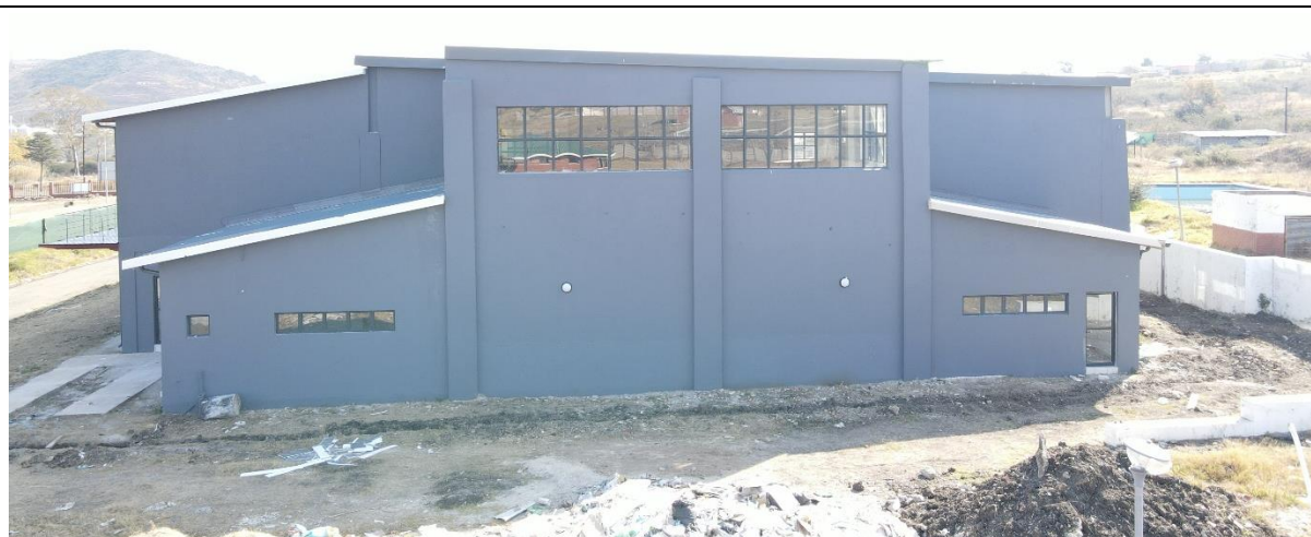
Side View of the MPC Building. Construction of concrete paving of walkways, concrete drains and general landscaping around the building structure is required
