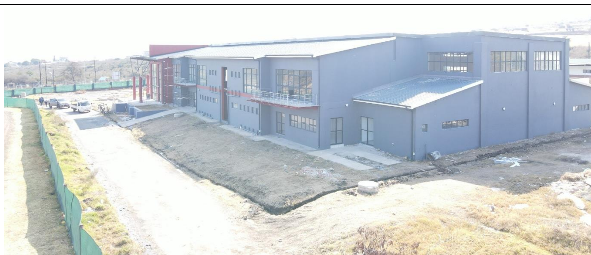
Side Front View of the MPC Building. Construction of concrete paving of walkways, concrete drains and general landscaping around the building structure is required
