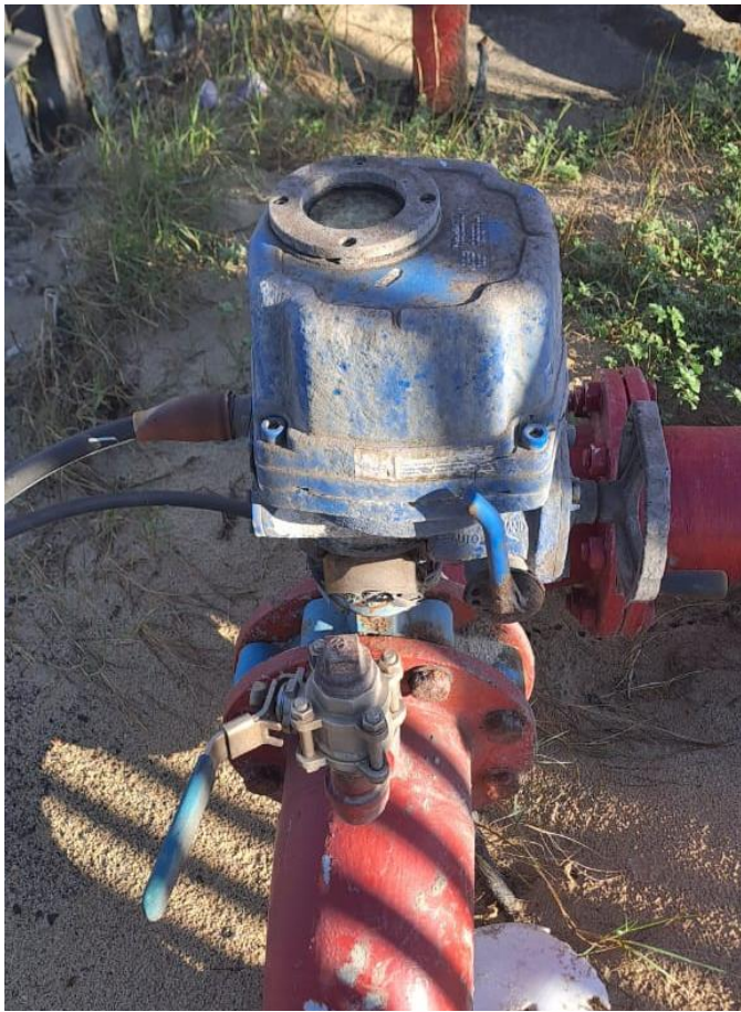
Figure 3: Actuator Valve
