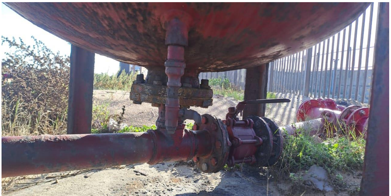
Figure 2: Valves to be replaced
