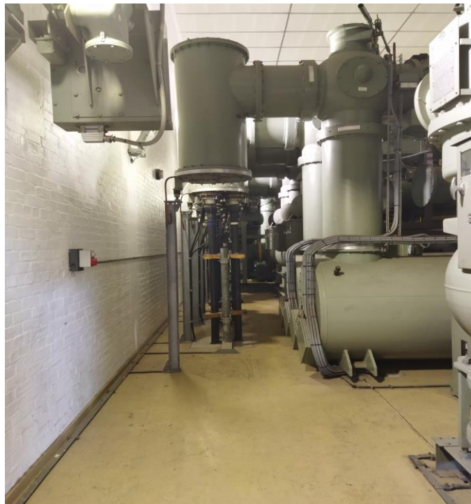
Figure 1: Vertical orientation of existing 132kV GIS termination
