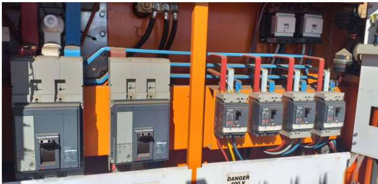
Figure 2 Existing mini-substation 400V compartment
