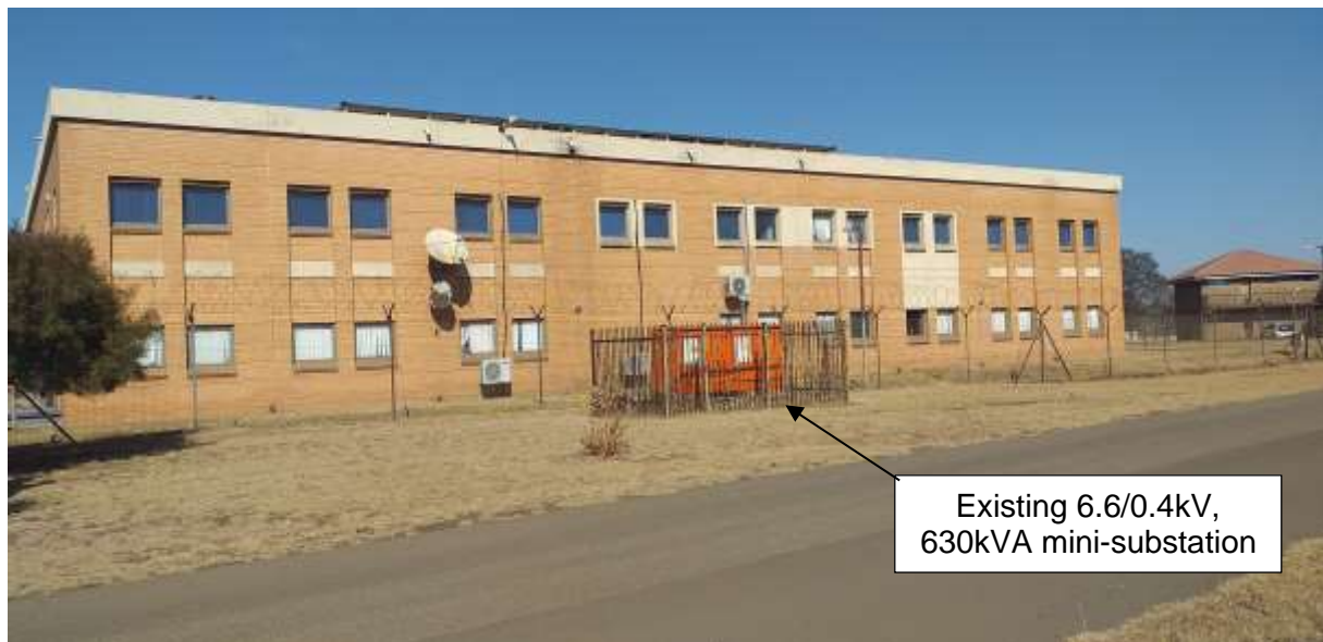
Figure 1 Existing mini substation to be used as a point of connection
