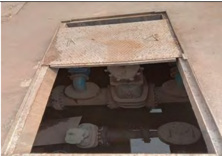
FIGURE 1 : WATER FLOODED VALVE CHAMBER.
