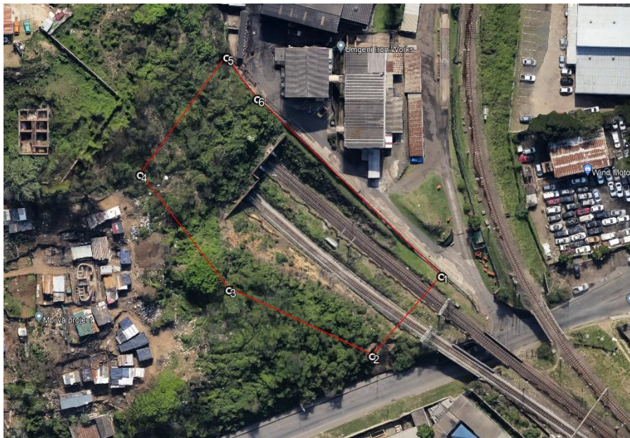
Figure 1 Umgeni Tunnel - Survey Area
