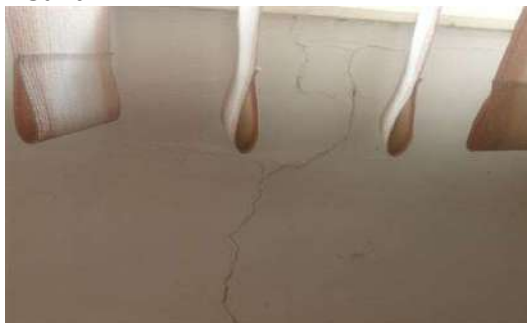
Figure 17: Vertical crack below the window sill - Stinah
