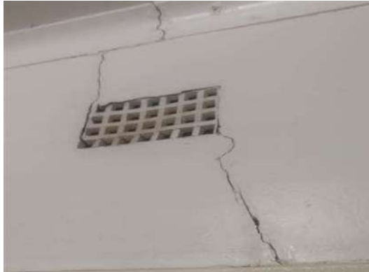
Figure 15: Vertical crack through the air brick - Stinah
