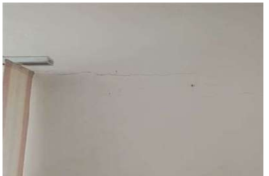
Figure 18: Horizontal crack at window edges - Stinah
