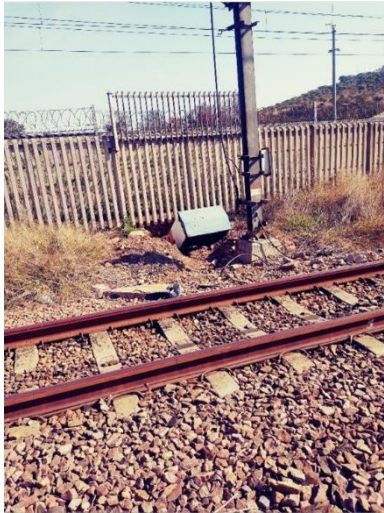
Figure 1: Shows under-dig breach
