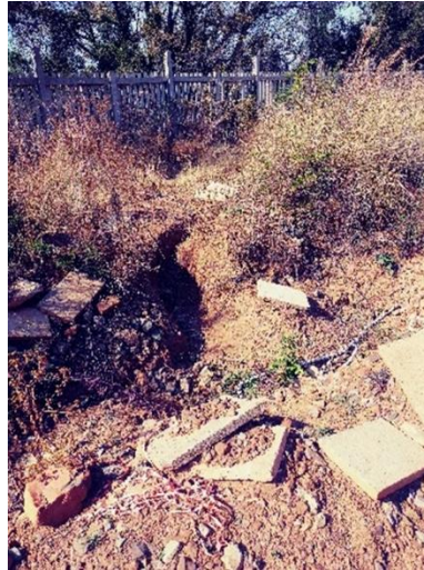
Figure 2: Shows illegal trenching due to cable theft.
