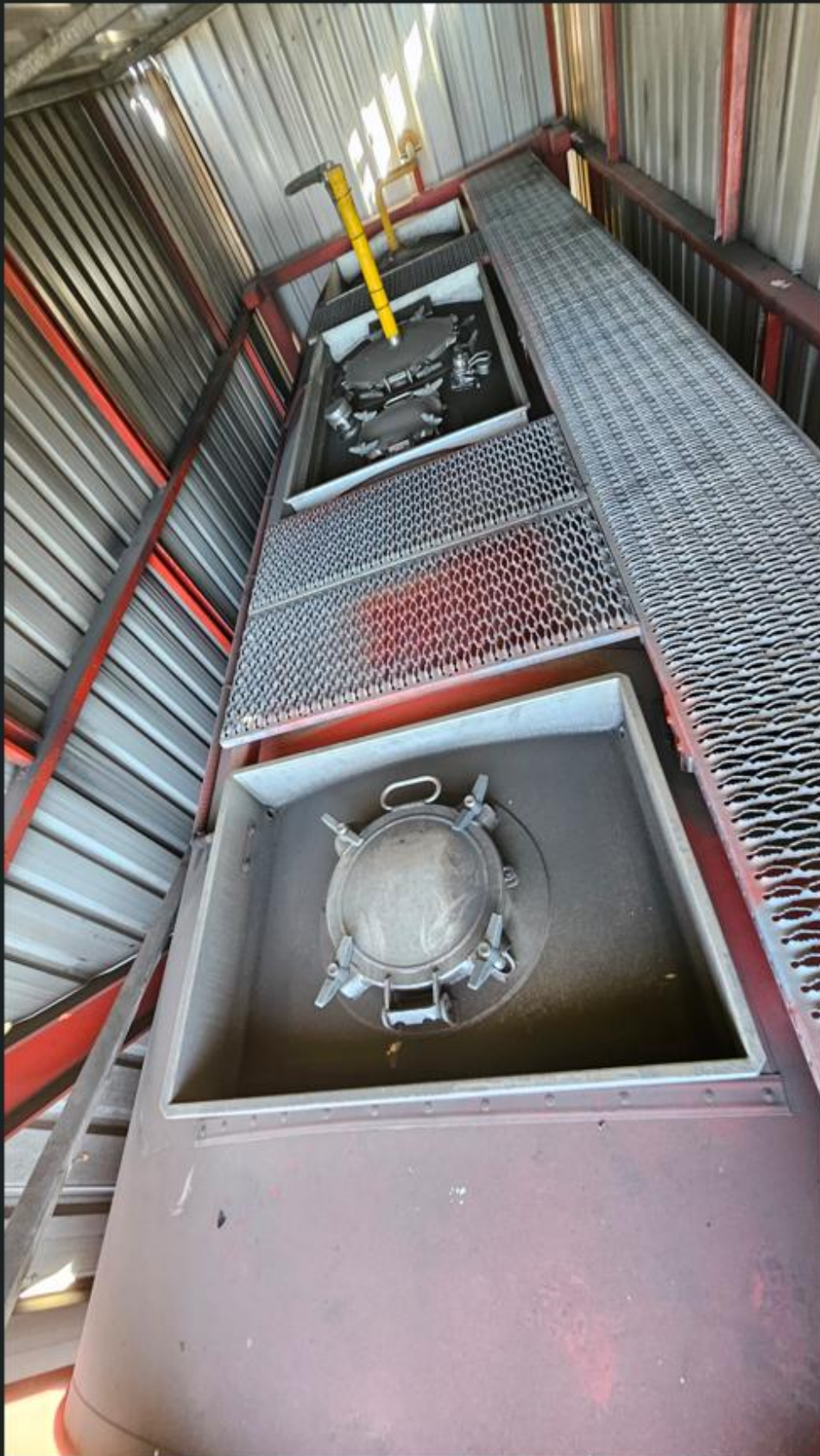
Mobile Bowser - Top of Tank View 1.jpg
