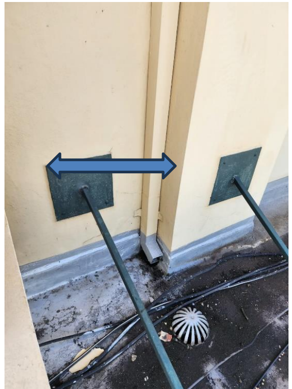
Photo 4: Steel tie-rods
