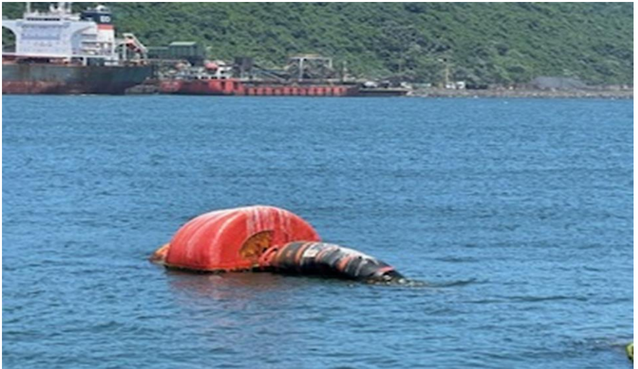
Leaking Coupling tomato-head: Require leak fixing, barnacle pressure cleaning, and re-greasing.
