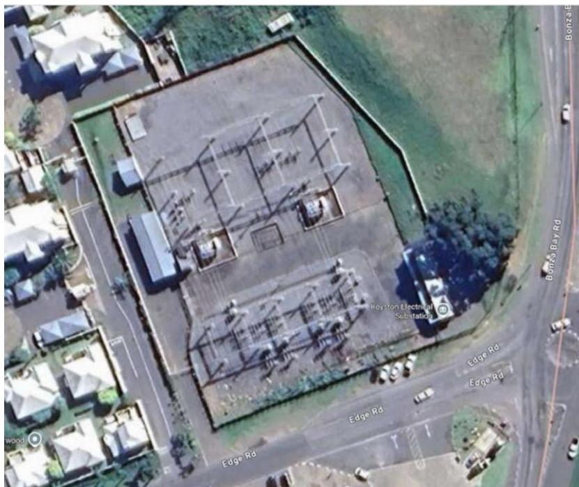
Figure 2: Example of a typical small Substation
