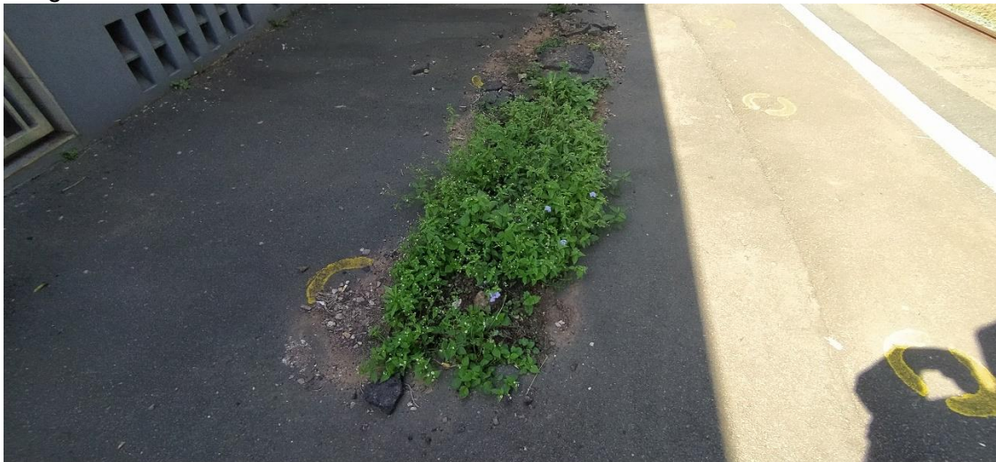
Image 4: Holes in Platform Tarmac
