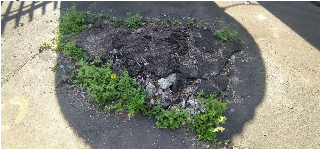
Image 3: Holes in Platform Tarmac
