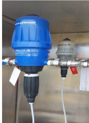
Chlorine Injectors
