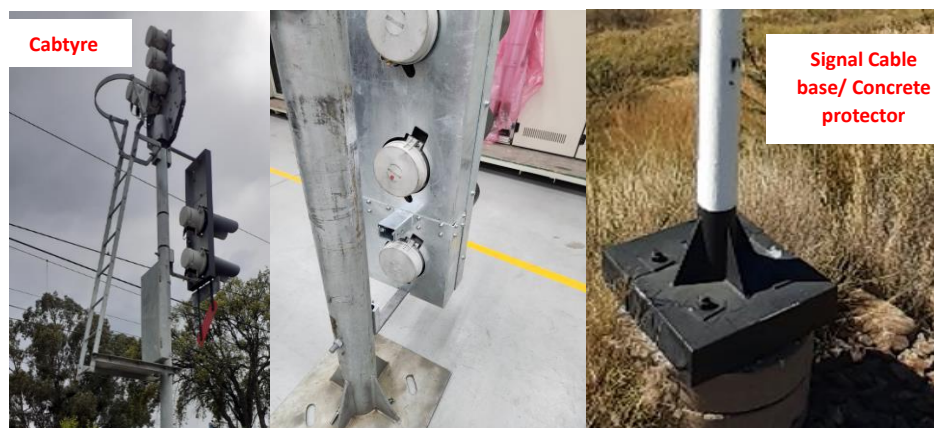
Photo 10: Signal: Signal Cable Base/ Concrete Protector Bolt cover protection
