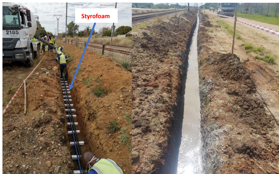
Photos 14: Cable trench with concrete mix
