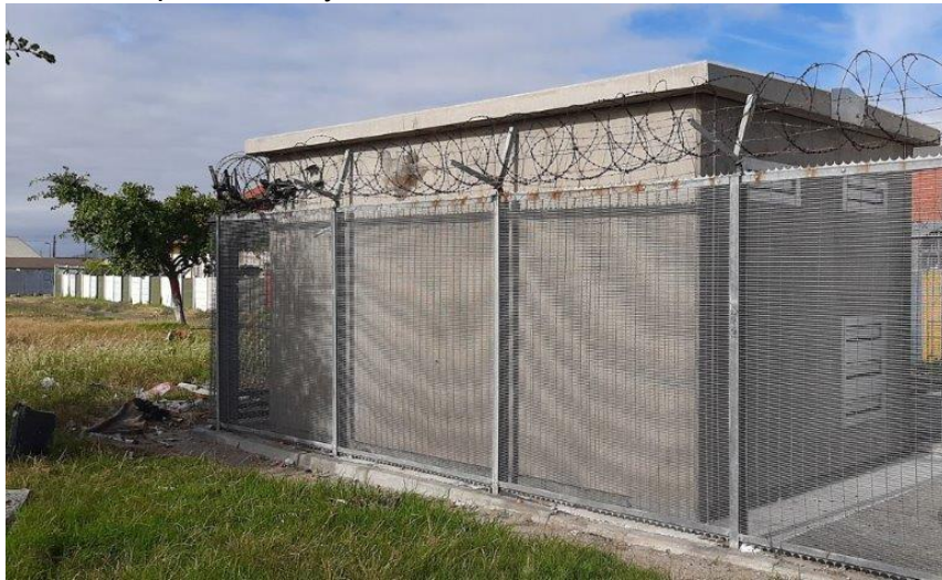
Photo 5: Bunker type solution Equipment / Apparatus Room example – note fencing.
