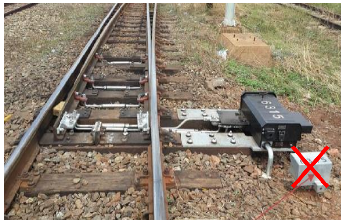
Photo 8: Points Machine requires a reinforced Lid & elimination of Junction Box
