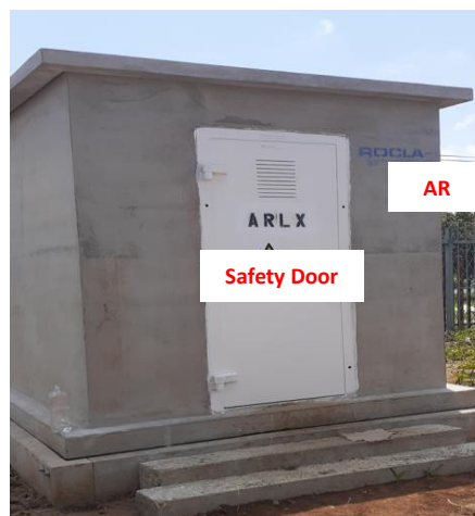
Photo 3: Apparatus Room type proposal with reinforced concrete
