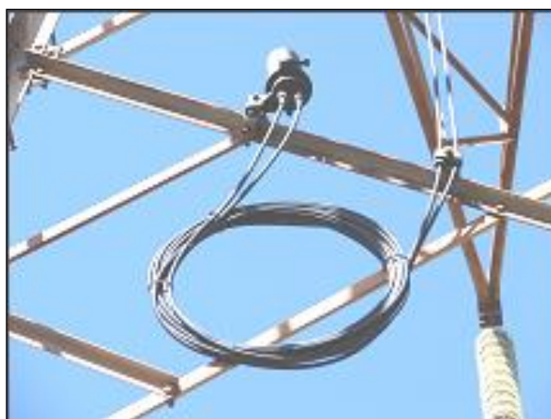
Figure 10: Dome Joints
