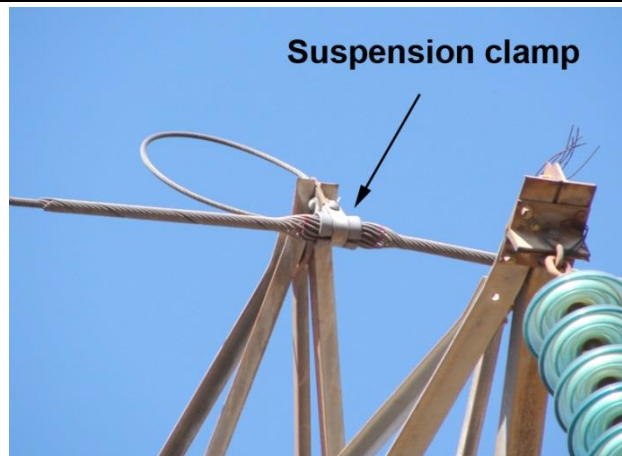
Figure 1: Suspension Clamp
