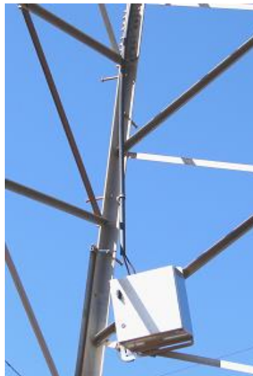
Figure 6: Joint Box
