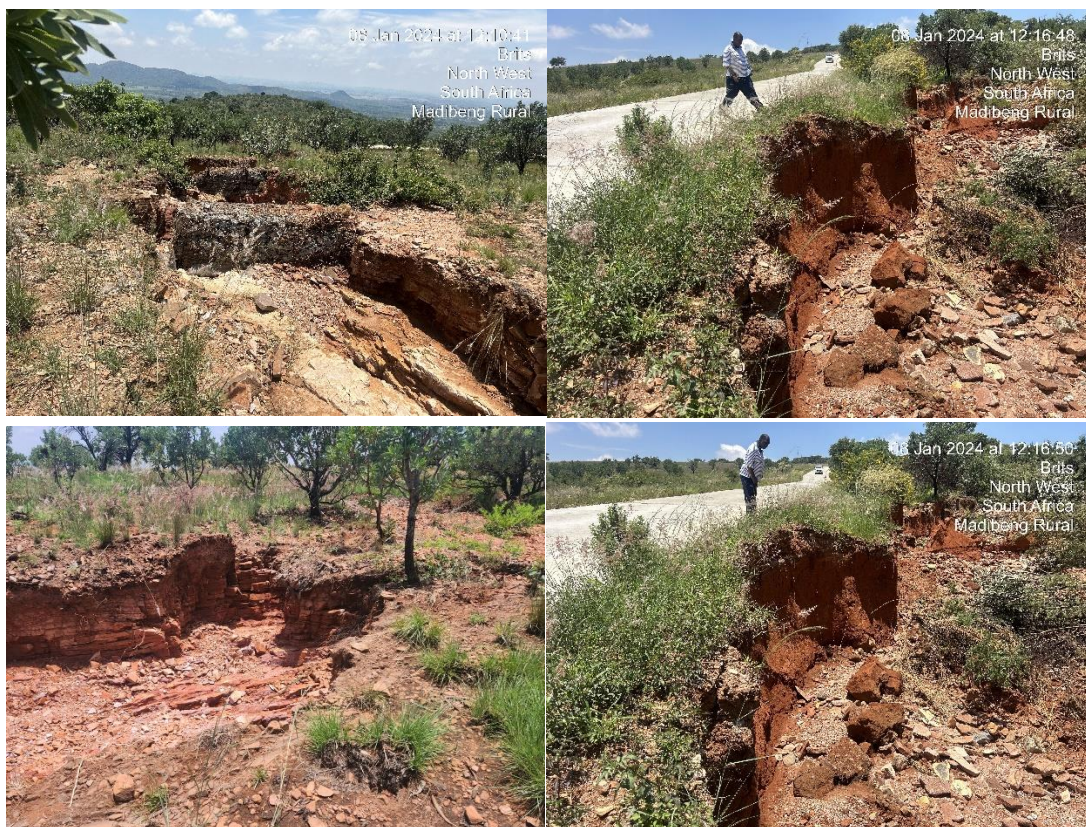
Fig1.1.1 Pictures showing the soil erosion impact onsite.
