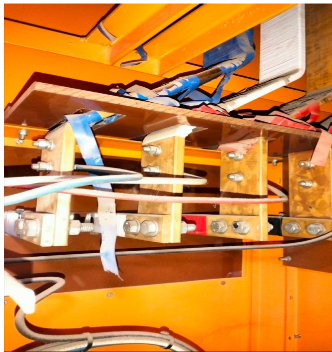
Figure 4: Main Busbar Arrangements
