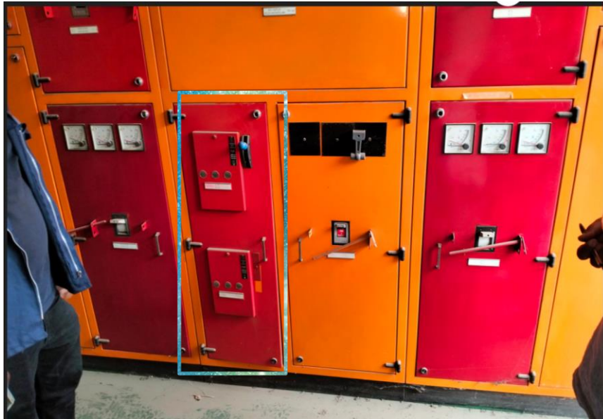
Figure 3 a : Funtional Unit for Retrofitting MCCB for RHF Plant
