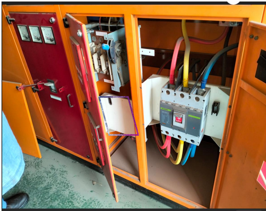
Figure 3 b: Opened Functional Unit showing chassis plate for mounting MCCB
