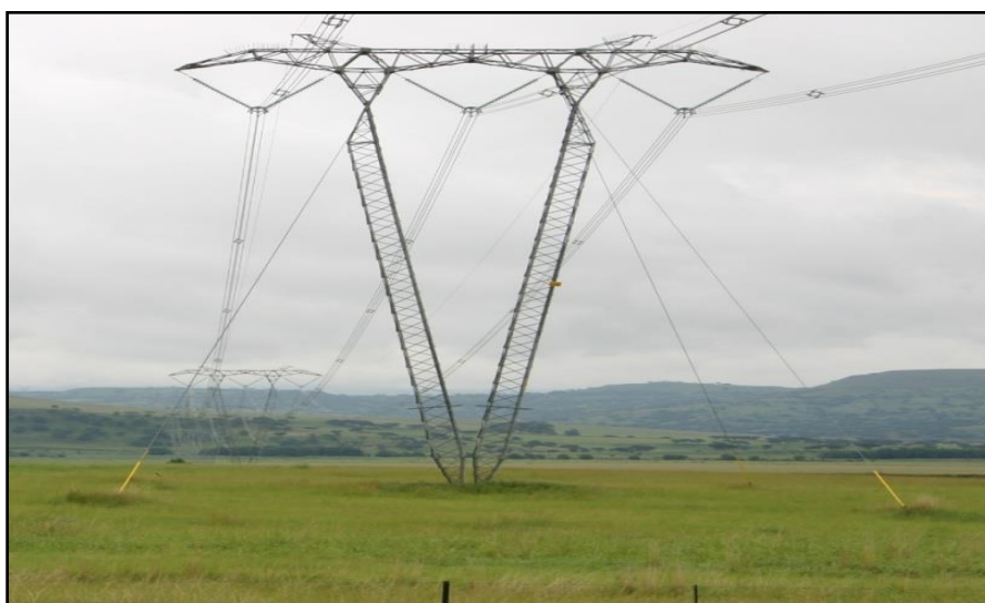
Figure 2: Guyed-V Suspension Tower
