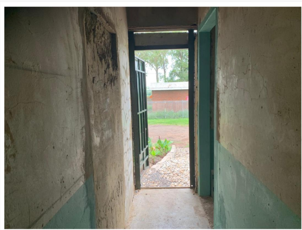
Uneven plaster and aging walls.
