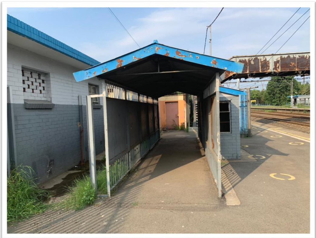
Broken window panes, and aging fascia boards.
