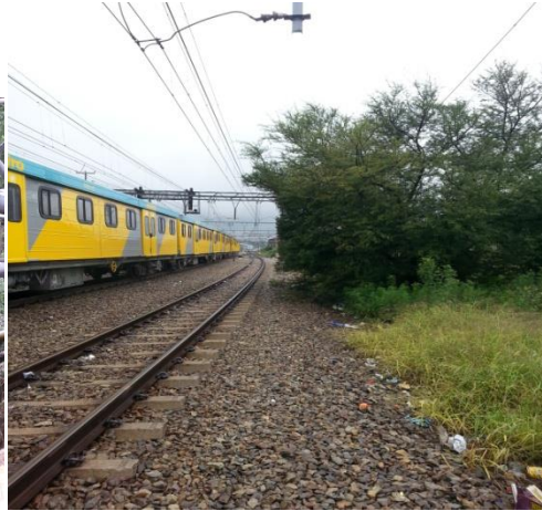
Fig 2.2: Trees encroaching on railway lines
