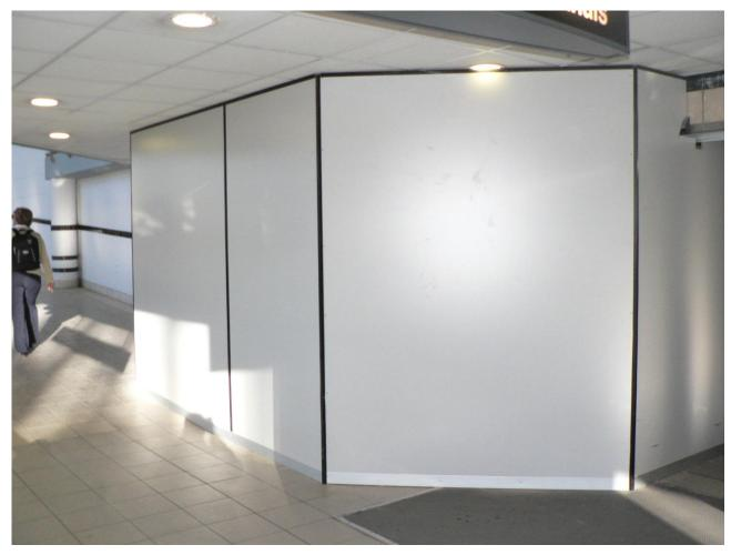
This type of hoarding is made out of 2100 h X 900 w melamine faced (Grey Cambrink) chipboard panel on metal supports. Generally, it will consist of four to six panels that can be placed around a particular area for maintenance or repair to floors.
