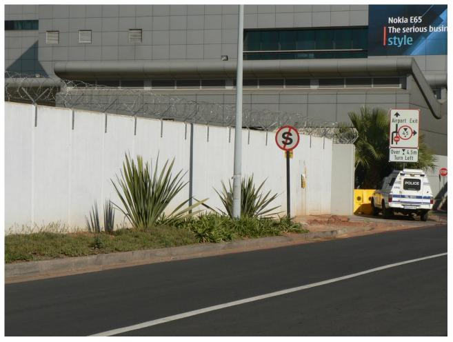
These are concrete panels 2100 h X 1500 w X 200 thick similar to the concrete walls around the airport site
