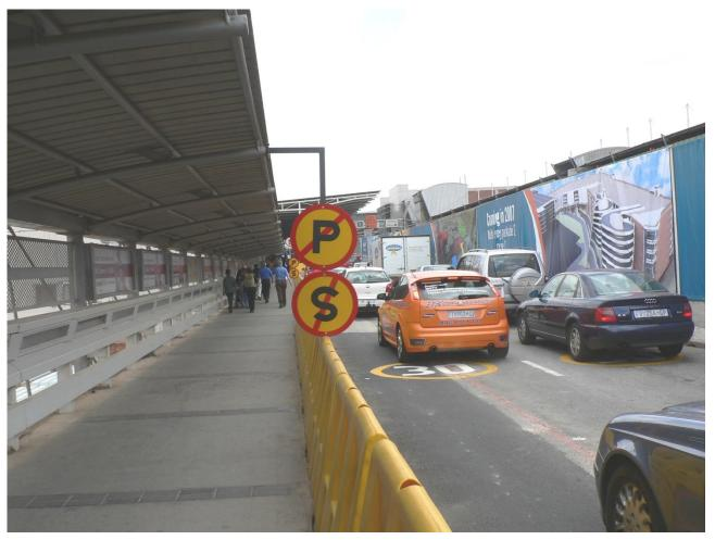
Yellow New Jersey barriers or orange plastic netting (at the discretion of the ORTIA-Project Manager) must be used to barricade the construction site from the public prior to construction work taking place.
