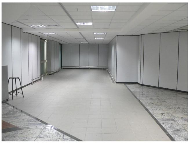
This type of internal hoarding will be applicable where construction work takes place adjacent to other tenants to minimise noise, dust and visual screening.
