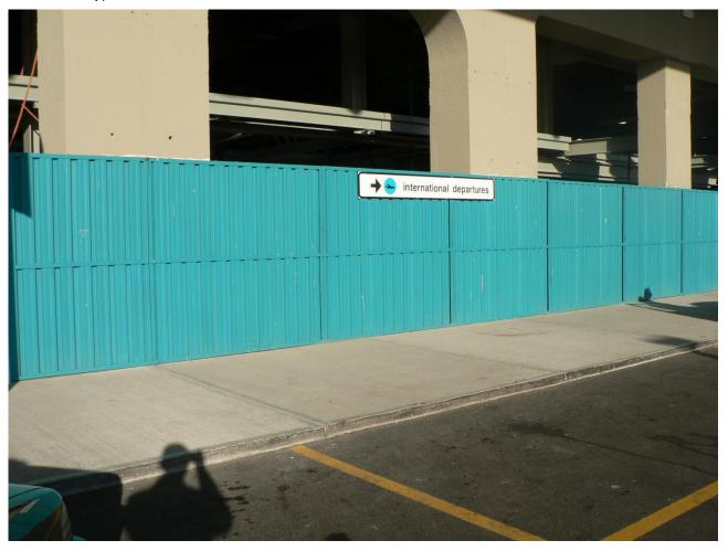
The sheet metal hoarding must be a minimum of 2000mm high around the perimeter of the construction site establishment. (See detail B)
