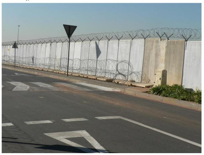
Pre-cast panel and pole hoarding will be used when indicated by ACSA. This hoarding will be used for contractor yards that will be used for extended periods of time. Specifications to be confirmed by the ACSA Project Manager.
