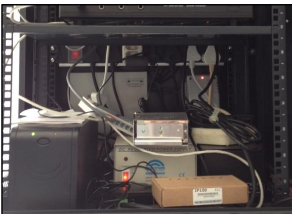
Figure 7: Example of Poorly Organised Security Equipment Cabinet
